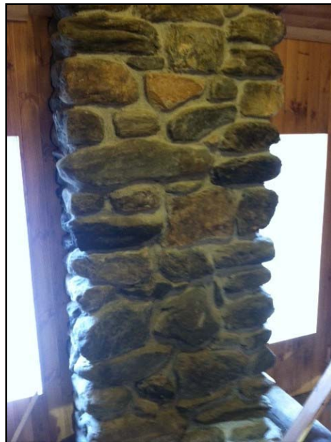
The historic stone fireplace and chimney are being carefully restored, with the original stones placed back into their historic locations.
