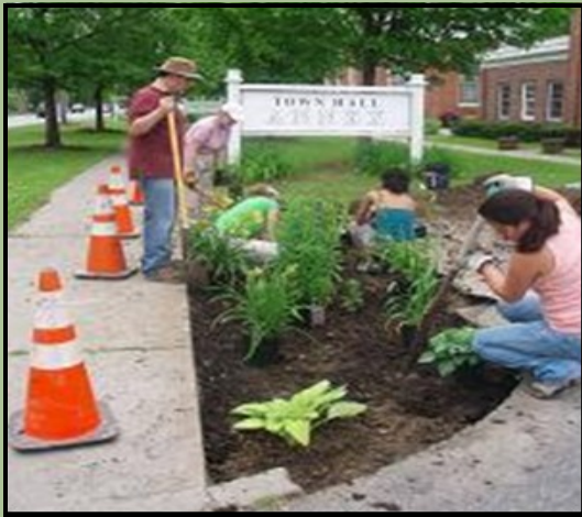
Rain garden during construction in 2009
