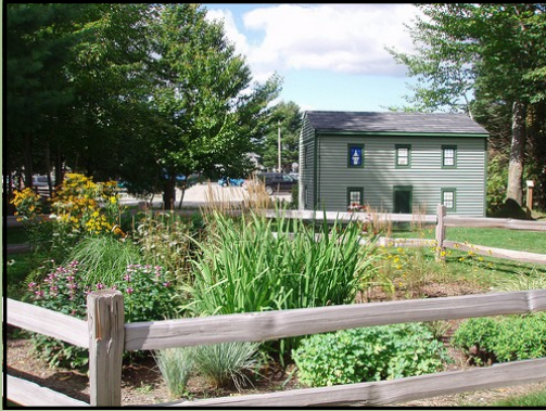
Smugglers Notch Resort demonstration rain garden in Jeffersonville was constructed in 2007. This rain garden captures runoff from two paved surfaces and is a part of a 'Where Does the Water Go?' tour of the Resort's stormwater management sites.
