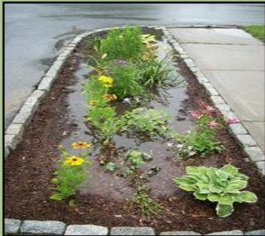
This 120 sq. ft. rain garden captures and treats stormwater runoff from the Town Annex parking lot. It is also designed to serve as an educational demonstration project
