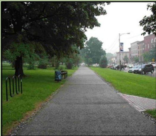
Taylor Park porous concrete sidewalk
