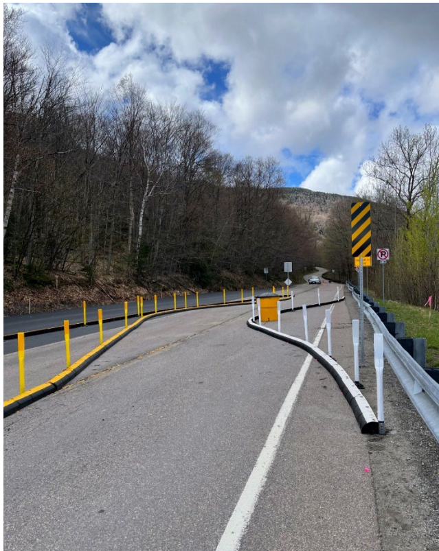
A Newly Installed Chicane
