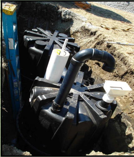
Installation of the two underground cisterns for stormwater storage
