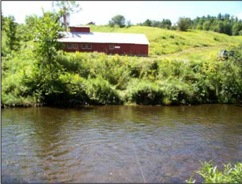
M04-B is a transitional segment between a very broad and semi-confined valley (B type channel)
